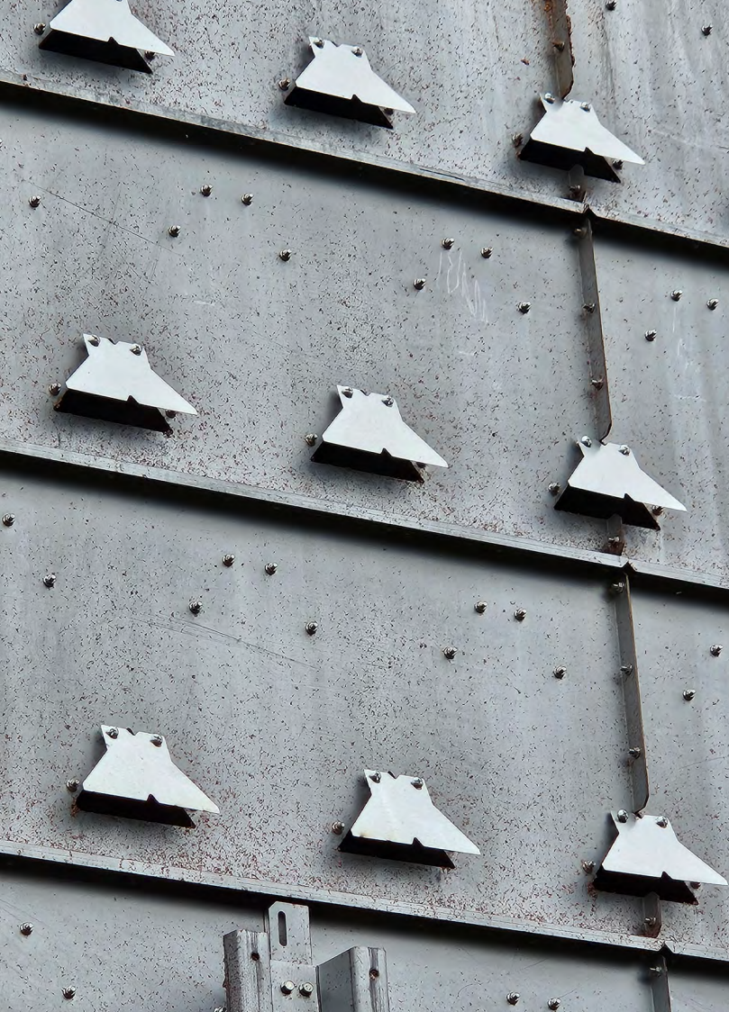
Duct covers open while dryer running
